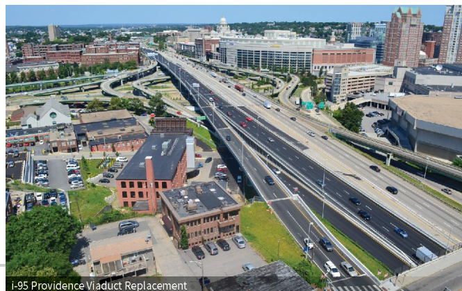
I-95 Providence Viaduct Replacement
